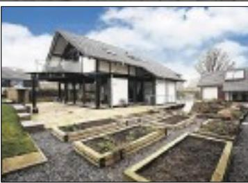
**GOING DEUTSCH:** The shell of the house was pre-fabricated in Germany but the fit-out, eco-additions and landscaping were done by owners Rod and Maureen Kelly. Cumberworth Lodge is highly insulated and ground source heat pumps and solar panels further slash the energy bills.
